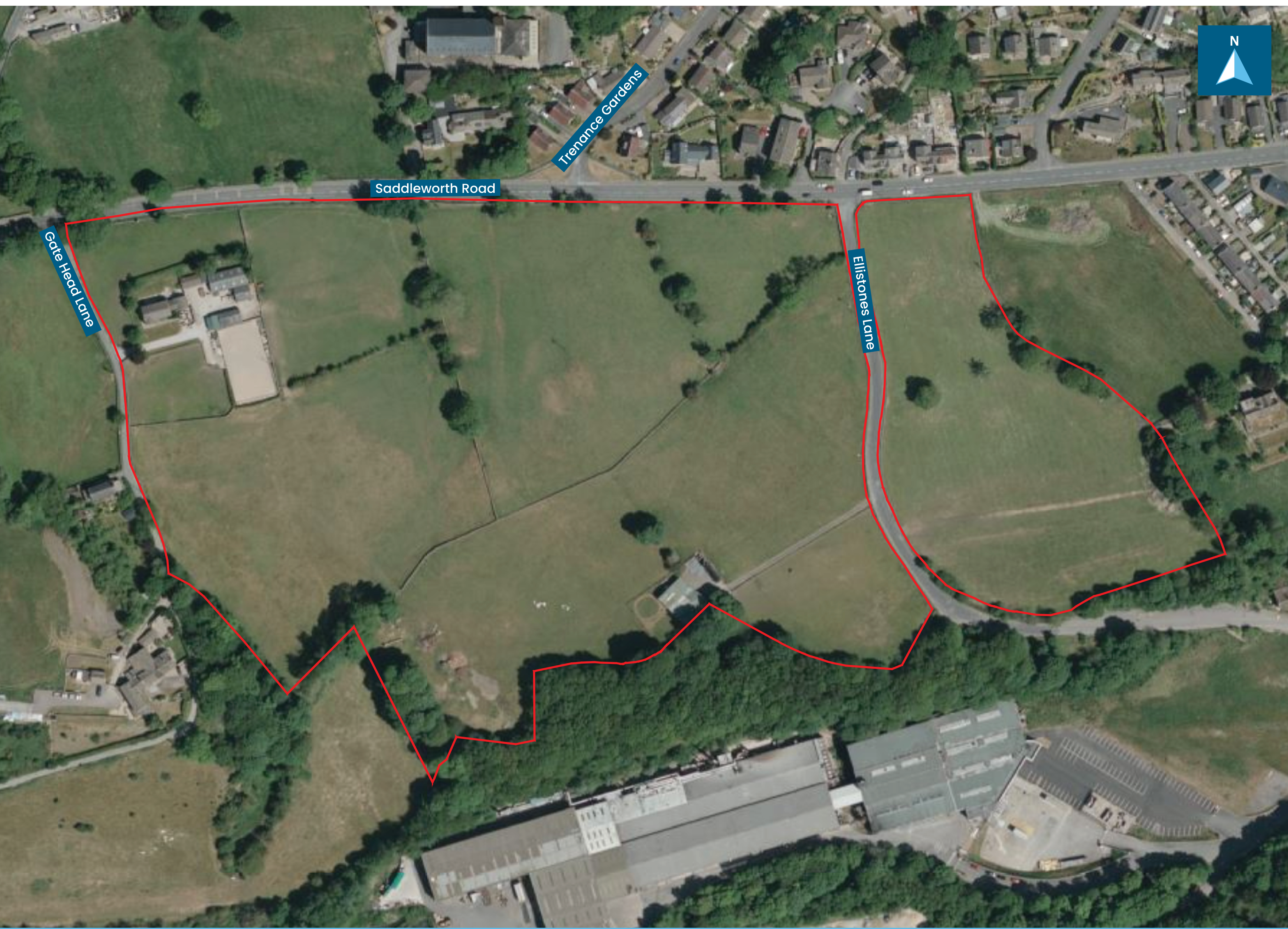
Aerial view of our site at Ellistones Gate, Greetland
